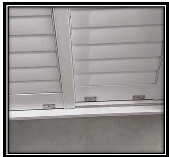
Back of panels – Bottom wheels
